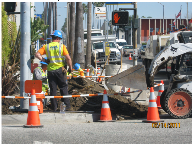
Installing Fiber and Conduit
