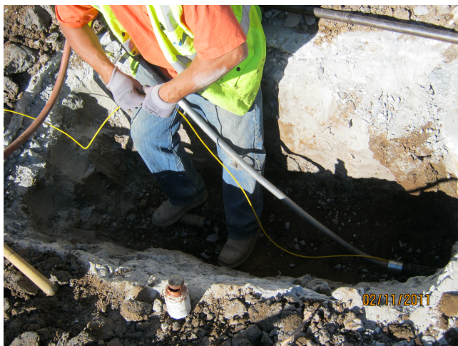
Working with conduit in a trench.
