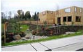
At Shamrock Heights, Cam West Development combines a traditional feel with innovative stormwater methods. Reuse of high-quality site soil, plus mulching, support a vibrant landscape.
