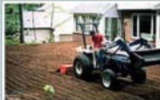
On many sites (here in a Snohomish home remodel) it is more cost effective to till compost into the existing soil. Tilling 2-3 inches of compost into any soil - sand, clay or till - makes planting easier and grows a healthier landscape.
