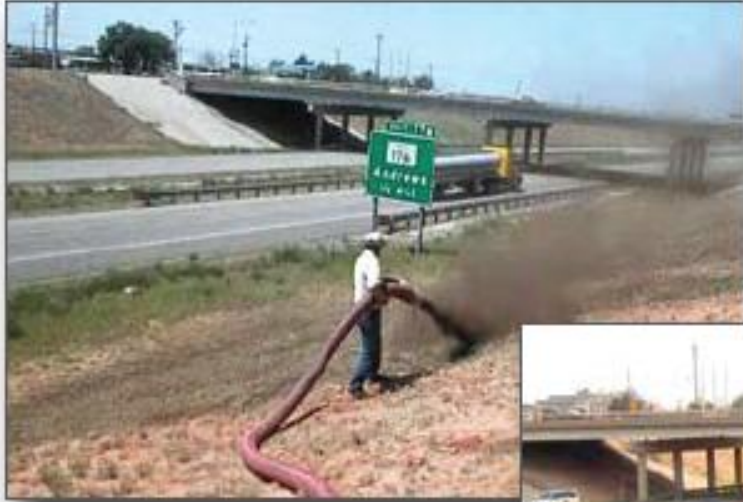
Applying a compost blanket on a bare and eroding slope
