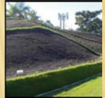
Slope Protection and Erosion Control Blanket
