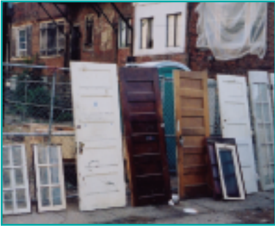
Tiles (top) and doors (bottom) were recovered from the 2003 West Philadelphia deconstruction pilot project, and were sold to local markets.
