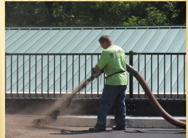
MCS Inc. worker installing growing media made from compost on green roof. www.mcsnjinc.com
